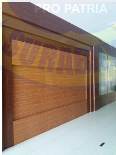
Gambar 4.4 Pekerjaan Alumunium Composite Panel finish garda pintu lift
