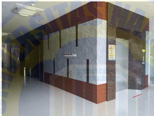
Gambar 4.3 Pekerjaan Alumunium Composite Panel finish garda pintu lift
