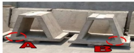
Fig. 11: Precast Foundation Design A & B
