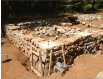
Fig. 1: Implementation of stone foundation
