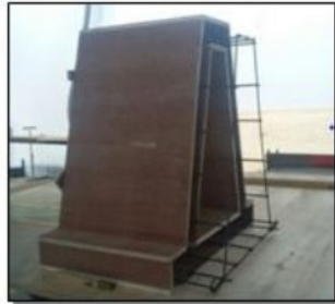
Fig. 6 : Formwork precast and wire mesh A model
