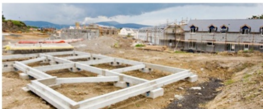
Figure 3. Precast foundation in Indonesia [13]
