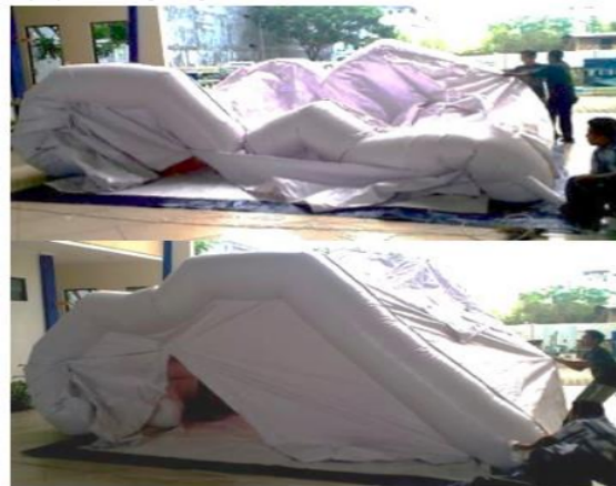
Fig. 1. Setting-Up Process of Inflated Portable Structure
