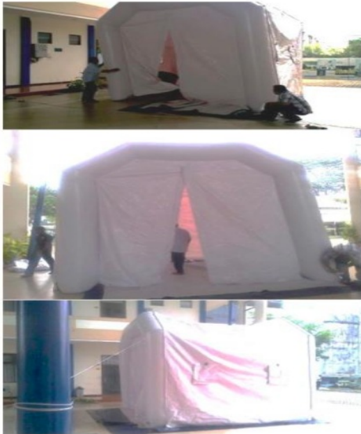
Fig. 2. Finishing Build-Up of Inflated Portable Structure
