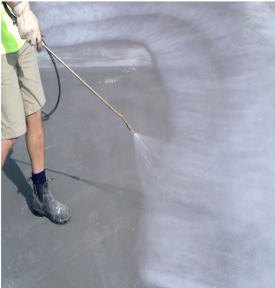
Gambar 3.2 Curing spray
