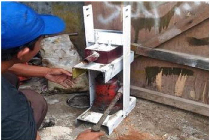
Gambar 7.2 Proses Pres Paving Block
