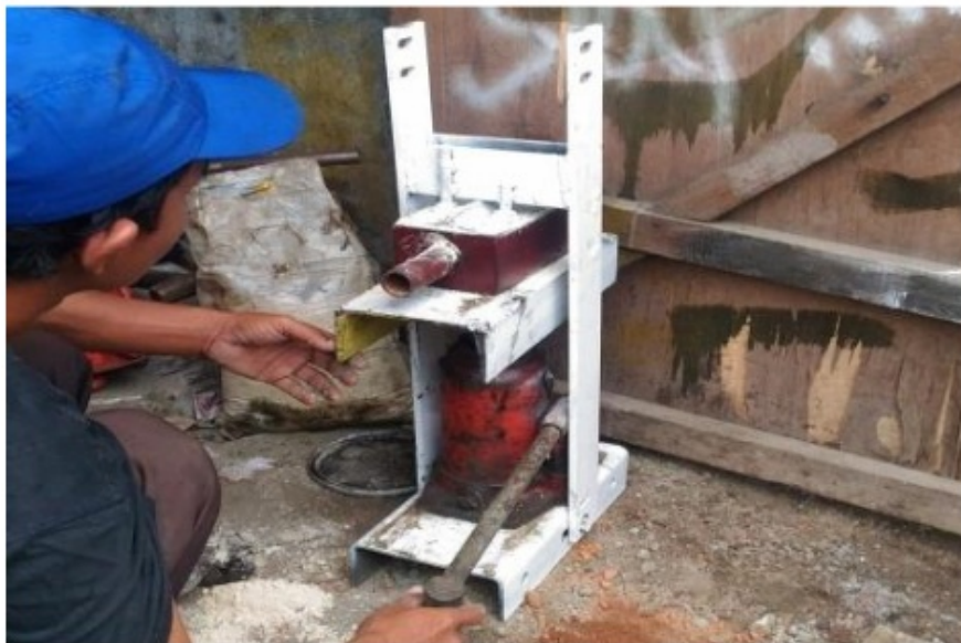
Gambar 7.2 Proses Pres Paving Block
