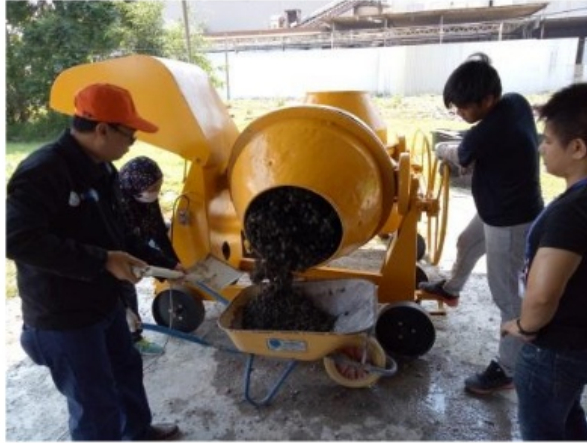
Gambar 6.8. Mixing pengecoran
