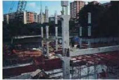
Multi-fixed precast columns
