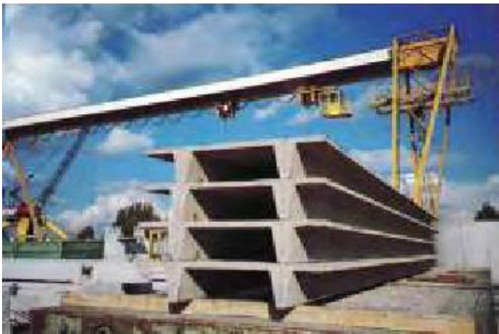
Gambar 1.7 Lantai Precast (Sumber: Architecture In Precast Concrete, Building and Construction Authority, December 1999, ISBN 9971-88-707-X )
