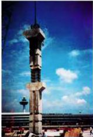
Precast columns, Changai Airport Terminal 2
