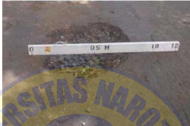
Gambar 2.13 Lubang ( Pothole )
