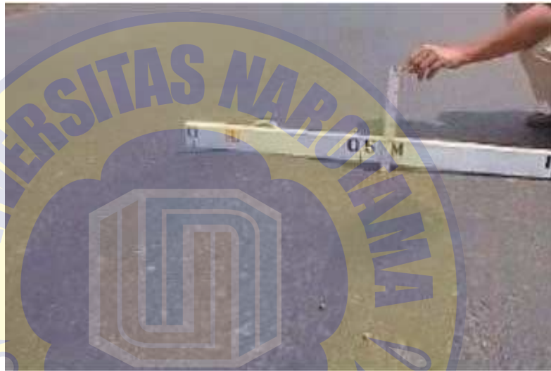
Gambar 2.15 Alur ( Rutting )
