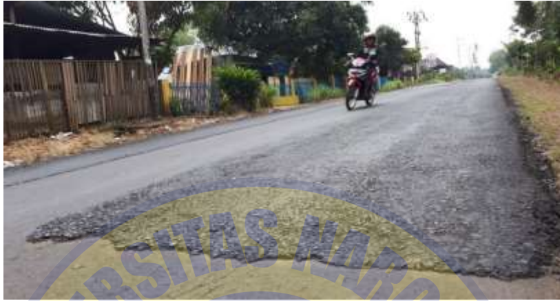
Gambar 2.11 Tambalan ( Patching and Utility Cut Patching )
