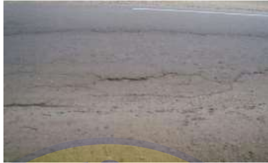
Gambar 2.4 Cekungan ( Bumps and Sags )
