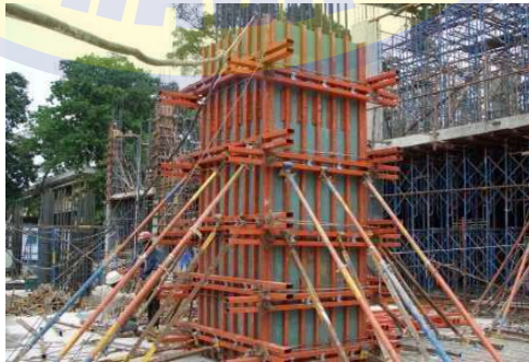
Gambar 2.1 Bekisting Semi Sistem
