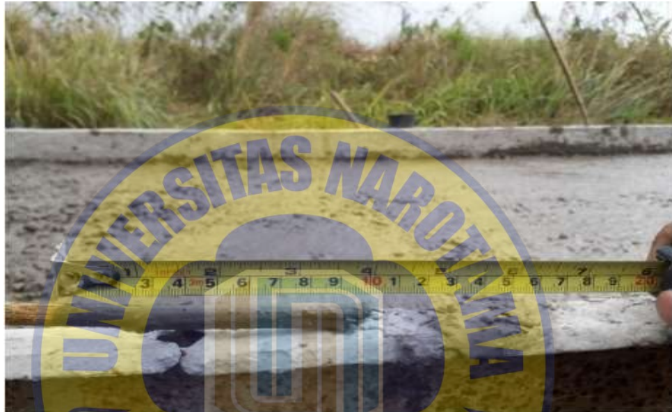
Gambar 4.9 Ketebalan LC (Lean Concrete)
