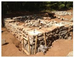
Fig. 1: Implementation of stone foundation source:http://www.thiscobhouse.com/wpcontent/uploads/2013/08/IMG\_0791-1024x768.jpg
