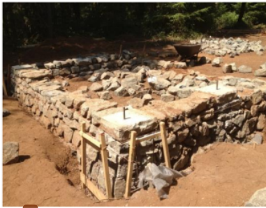
Fig. 1: Implementation of stone foundation
