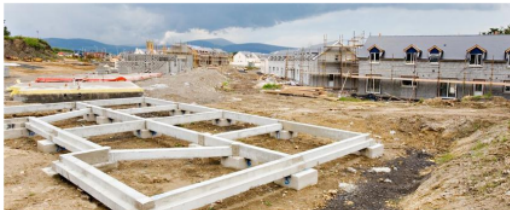
Figure 3. Precast foundation in Indonesia [13]
