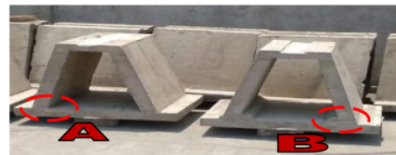
Fig. 11: Precast Foundation Design A & B
