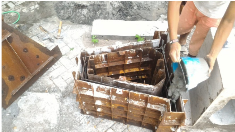
Figure 2. Trapezoid A Model Foundation in Progress
