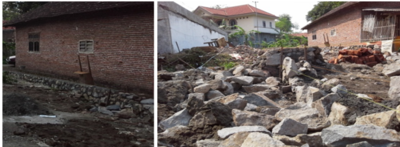
Figure 1. Stone Foundation
