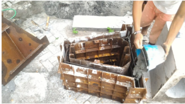
Figure 2. Trapezoid A Model Foundation in Progress
