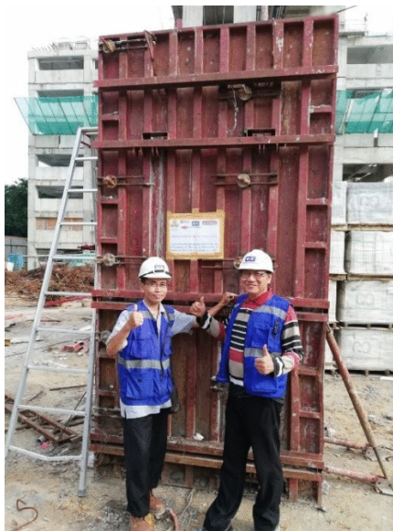
Figure 5. Mock-up form with the size of 1000 x 1000 x 2500 mm 3 .
