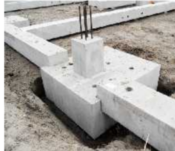
16 Fig. 2 Precast foundations
