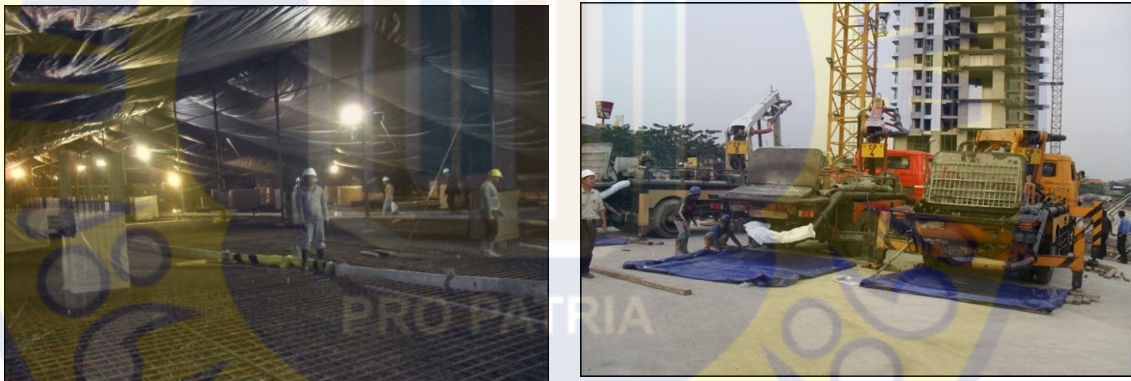
Gambar 4.12. Proses pengecoran mass concrete
