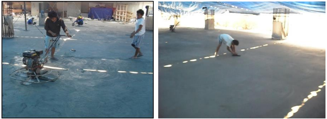
Gambar 4.13. Proses trowel floor hardener
