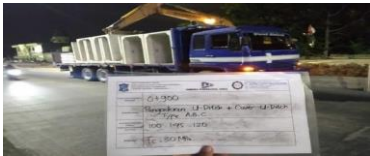
Pengadaan U-Ditch + Cover U-Ditch Uk. 100.145.120 fc 30 Moa Pabrikasi
