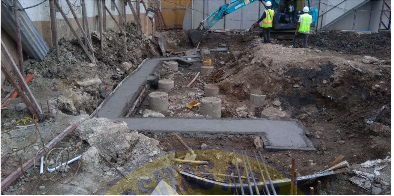
Lampiran 24. Tampak Capping Beam Soldier Pile
