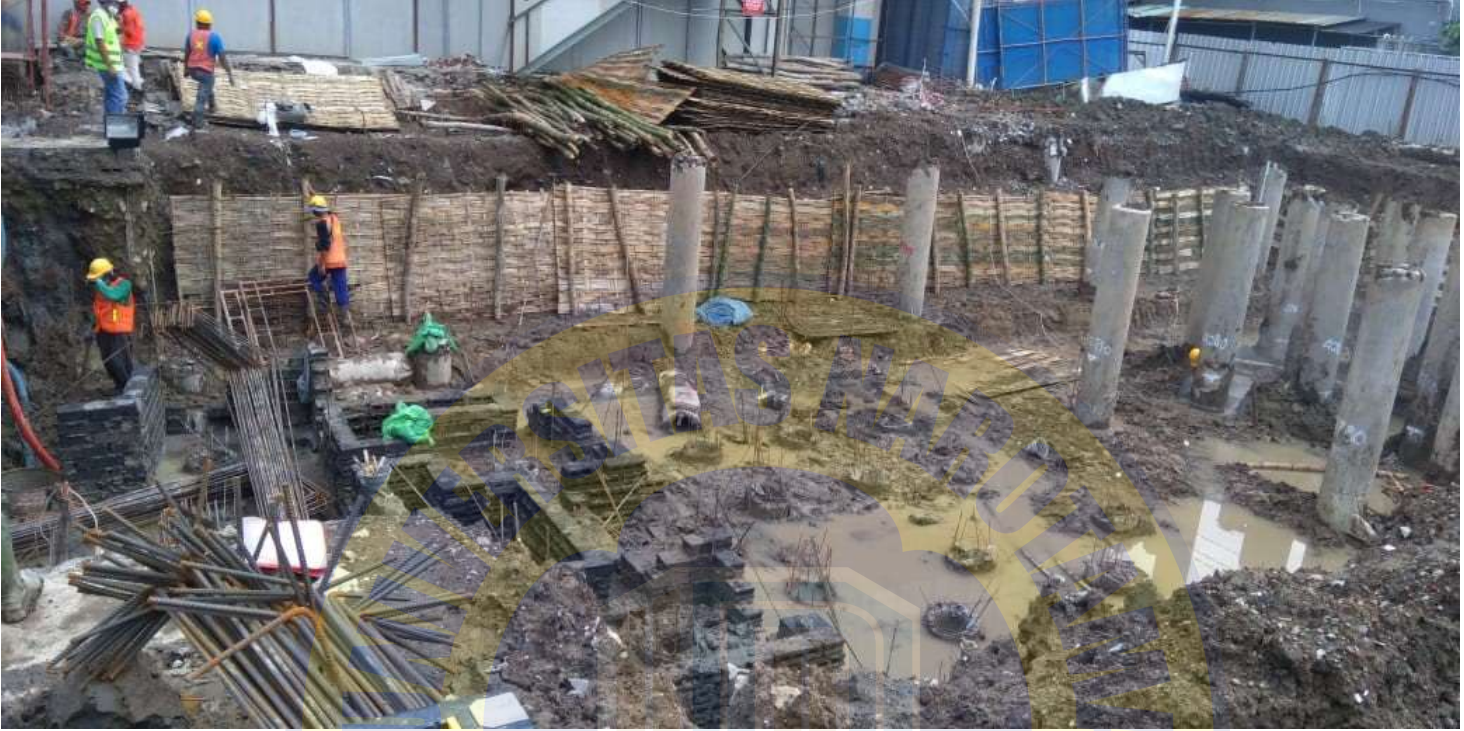
Lampiran 22. Proses Dewatering Area GWT
